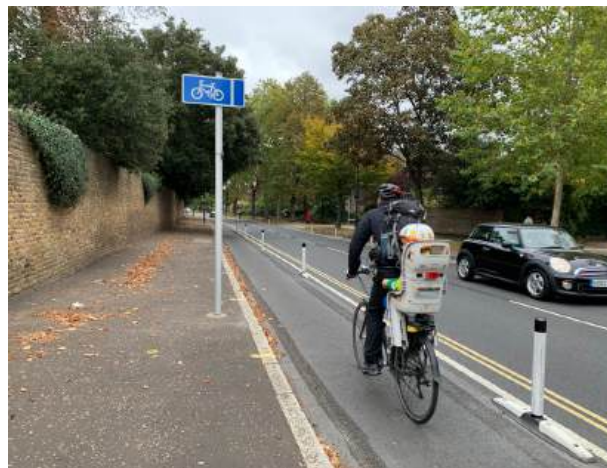
Light separated with-flow cycle track using wand-orcas.
