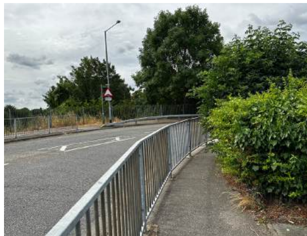
Footways narrowed by vegetation, street clutter, pavement parking or unnecessary guard rail.
