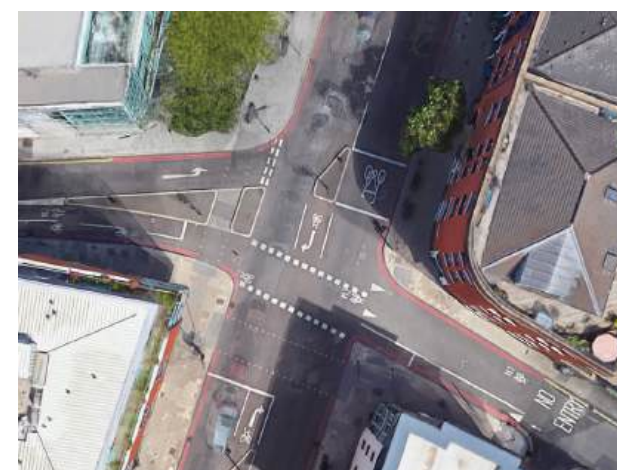
Signalised junction with pedestrian and cycle parallel crossings.
