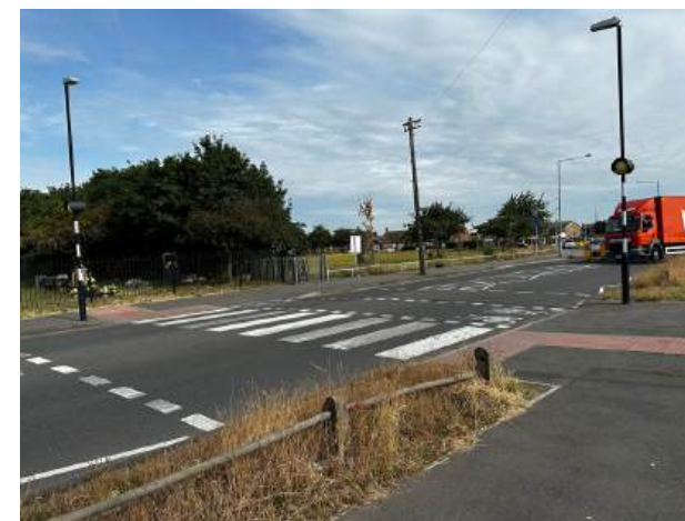
Existing parallel zebra crossing helps to link up walking and cycling routes.
