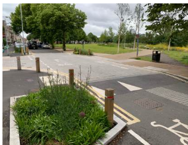
Raised table treatment in a low traffic environment.
