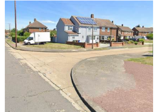
Side road junctions are very wide and lack dropped kerbs and tactile paving.
