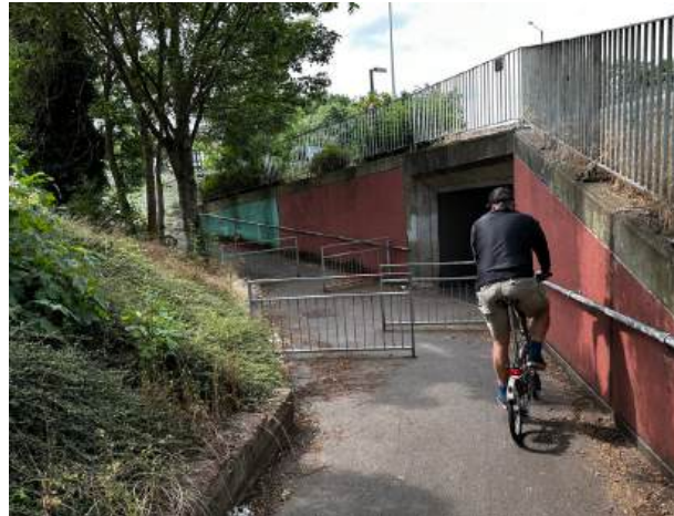
Poorly placed and designed barriers restrict people cycling and wheeling.
