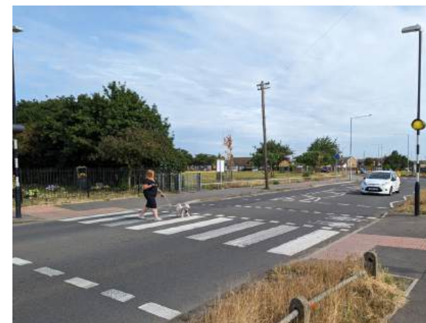
Parallel zebra crossings can help to connect up walking and cycling routes.
