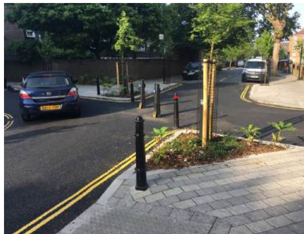
Diagonal modal filter with integrated tree planting and informal crossings.
