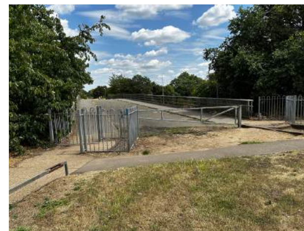
Some barriers can prevent access for people walking, cycling and wheeling.
